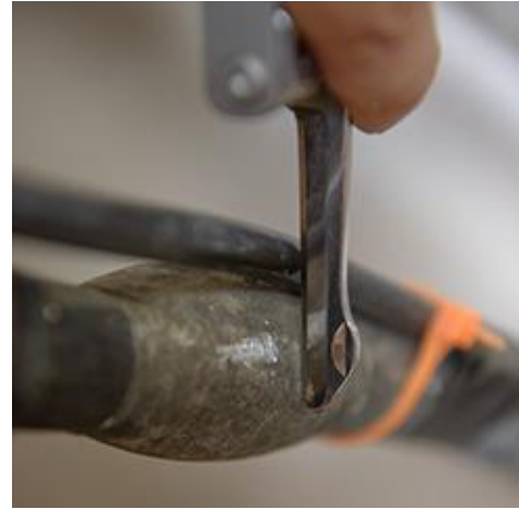
Figure 5: Wipe lead joint scratch test.
